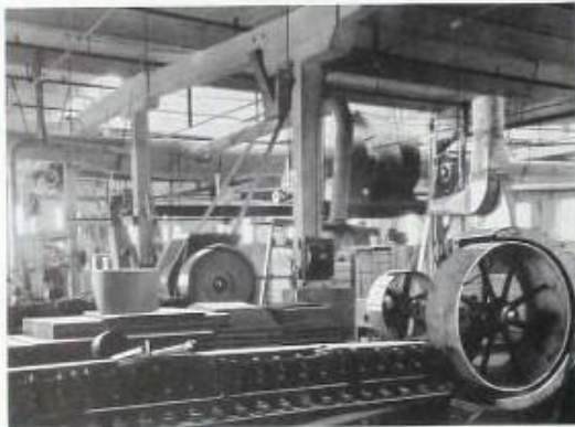
Sonora Plant, Saginaw, Mich. Woodworking, Exhaust System, "Sirocco" drive.
