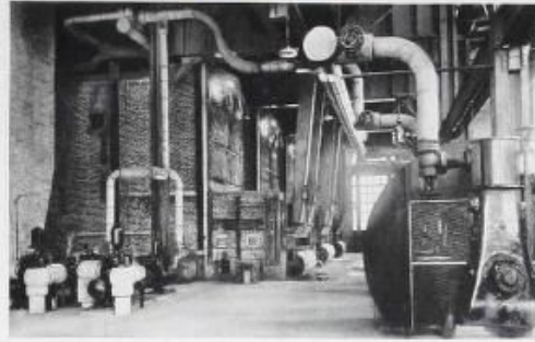
J. H. & C. K. Eagle Mfg. Co., Shamokin, Pa. Induced draft in boiler room with direct-connected "Sirocco" Fan and "A B C" Engine.
